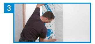
**Install a membrane strip** from 2 to 3 in (5 to 7.5 in) on the weather barrier.
