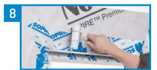
**Apply pressure on the membrane** using a hard roller for stronger adhesion.
