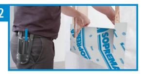
Apply the **SOPRASEAL STICK AVB AT** membrane on the lower part of the window and cover 5 cm to 7.5 cm (2 in to 3 in) of the weather barrier.
