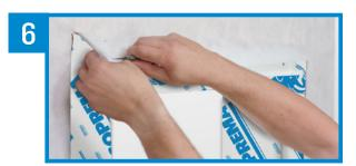
Fold the weather barrier membrane in place. Cut 1 in (2.5 cm) of the weather barrier to clear the metal flashing.
