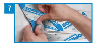
Seal the corners of the metal flashing with the SOPRASEAL STICK AVB AT membrane diagonally at each end.
