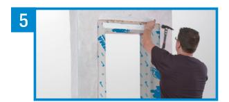
**Install the metal flashing** in compliance with the National Building Code.
