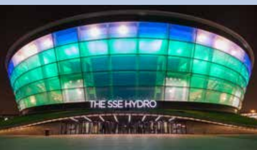
The Hydro Glasgow (Escocia) – Arqt. Foster and Partners
